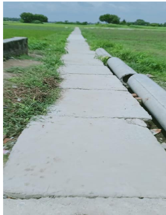
Drain constructed in Tilmapur village
